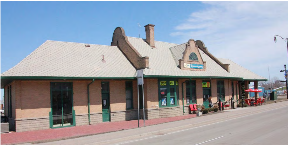
Figure 3-11: The Depot/White Earth Transit Station in Detroit Lakes
